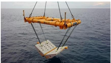
PCM lifted Flat to minimise load transfer induced embedment.
